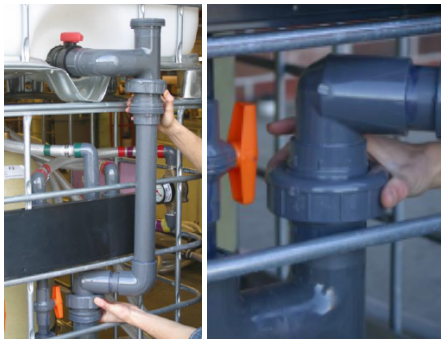
Figure 19 – Attach the Backwash Arm
