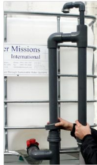
Figure 20 – Attach the Overflow Extension Assembly
