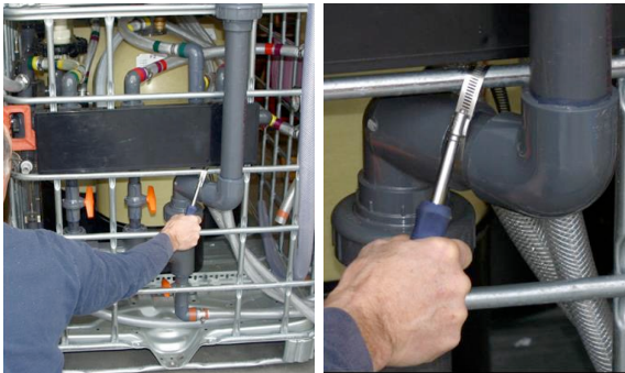
Figure 25 – Insert Hose Clamp to Support Backwash Arm
