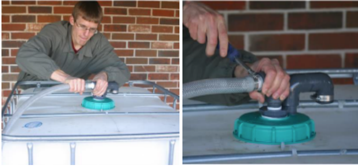
Figure 14 – Attach the Backwash Tank Feed Hose
