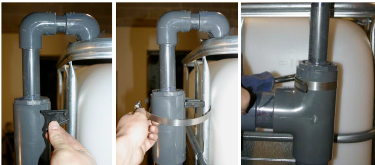
Figure 23 – Insert Spacer on Upper Overflow Extension
