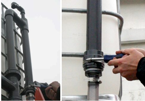
Figure 24 – Insert Spacer on Lower Overflow Extension
