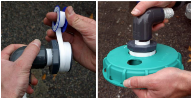
Figure 11 – Attach the Backwash Tank Inlet
