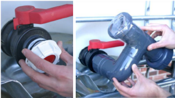
Figure 17 – Attach the Backwash Tank Outlet
