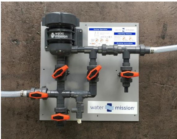
Figure 9 - Erosion Chlorinator Installation with Hose Connection
