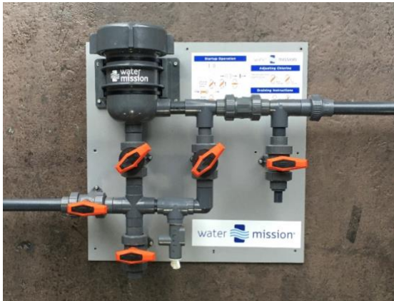
Figure 8 - Erosion Chlorinator Installation with Pipe Connection
