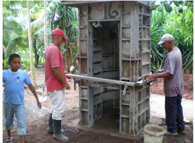
The provided aluminum forms are assembled and used as a mold for the concrete structure. A vegetable oil is applied prior to pouring the concrete, making it easier to release the forms once the concrete has set.
